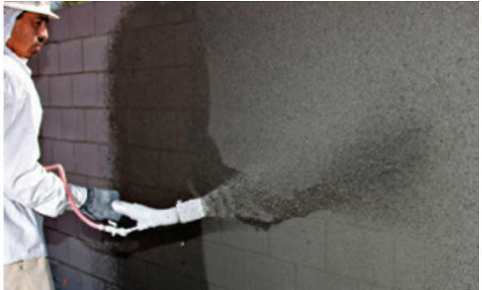
SPEC MIX FBC Stucco is engineered for gun-applied basecoat in one- and three-coat wall systems
