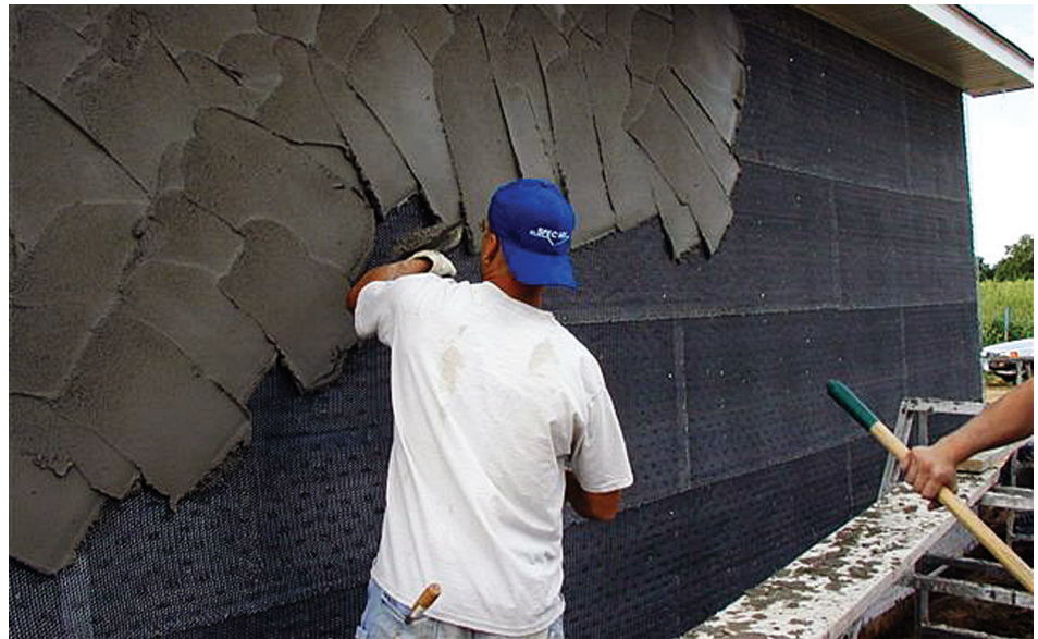
Application of proprietary, preblended, shrinkage compensated basecoat
